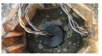
Step 4 - Install loops through black duct bung. DO NOT REMOVE THIS BUNG.
