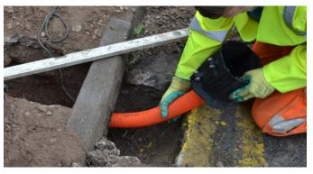
Step 2 - Duct is connected to spigot of loop box and surrounded with 150mm ST4 concrete.
