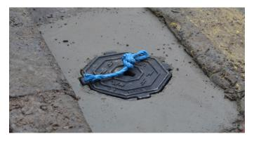
Step 3 - Top surface is applied ensuring loop box lid is flush with finished level.
