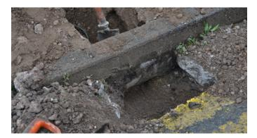
Step 1 - Entry to remote chamber is excavated and 50/100mm duct is installed.
