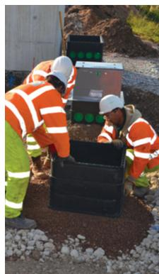
The NAL STAKKAbox™ Modula system is a range of thermoplastic, preformed twin wall, modular access chambers capable of withstanding vertical loads in excess of 40 tonnes without the requirement for any structural support. The chambers are easily adaptable on site to overcome services without any loss of strength, available in B, C, T and Loop chamber sizes for Motorway Communications installations.
