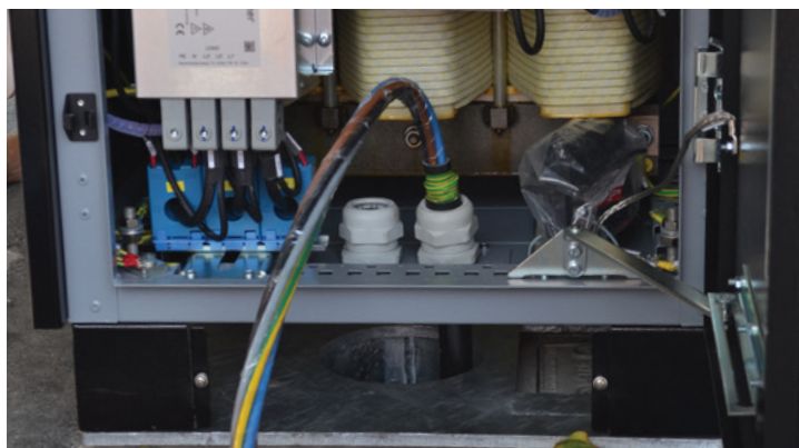
Step 5 - Lower the EV charge unit onto the Adapter Plate, using the locating pins to align. Ensure cable slack is being pulled through.
