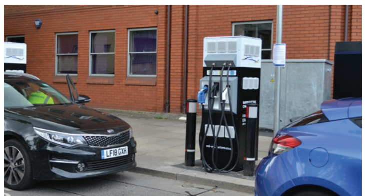
Step 8 - NAL X-LAST Standard protective bollards are installed into Retention Sockets leaving site operational, safe and futureproofed.
