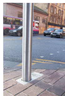
Block paviour using drop kerb wedge
