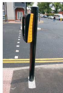
Black top installation without kerb wedge
