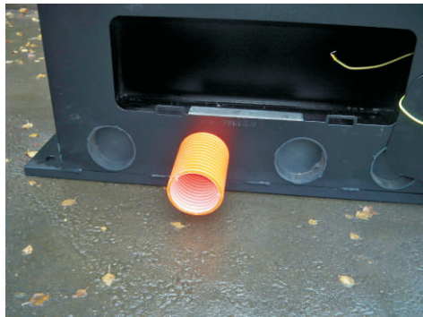
Positively connect duct
