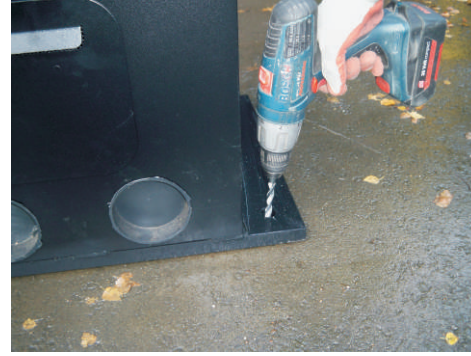
Drill 4 fixing points
