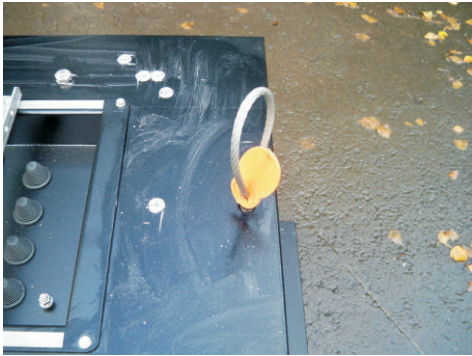
2 Lifting eyes installed
