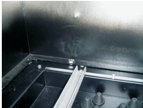
Position cabinet and bolt down
