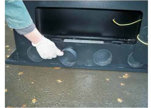
Remove required duct entry caps
