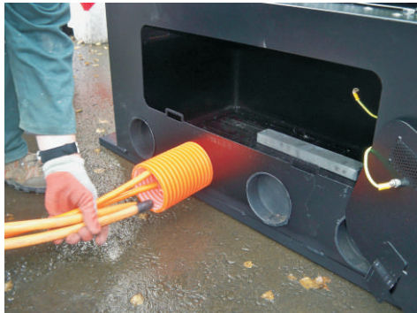
Cables can now be pulled
