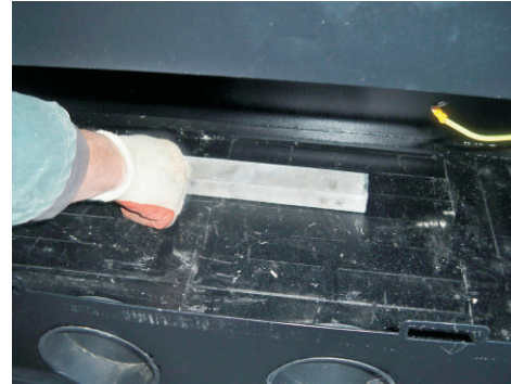
Extra ballast can be added if required
