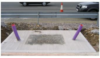
The NAL STAKKAbox™ ULTIMA offers a flexible access chamber system with no compromise on strength. Due to the design and the material used (Glass Reinforced Polyester Resin). This chamber can be used where a side-wall exceeds 1000mm and loading is a concern, making it ideal for A type Motorway Communication chamber installations.
