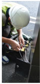
The Low Level Cabinet Base has been designed to simplify the installation, upgrading and replacement of all types of electrical control cabinets, where the overall height of the controller is crucial. The system offers a low level base plinth and gland tray with access to underground cables through a lightweight composite cover and frame situated directly in front or behind the cabinet.
