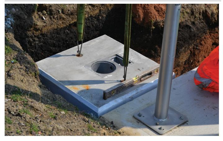
Step 3 - Lower Precast Foundation into the excavation using the pre-drilled lifting points, ensuring the orientation of the duct entry points are in line with the direction of the ducting. Connect duct if required.
