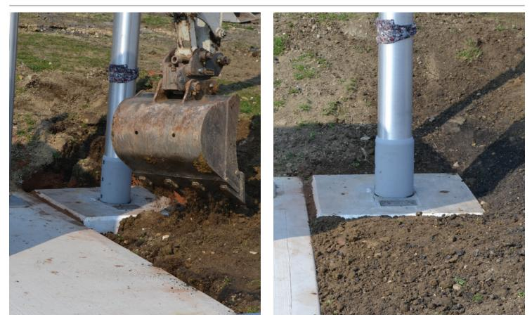
**Step 5-** Once the block is level backfill with dug material. Dug material must not contain pieces larger than 40mm. Alternatively use self-compacting material such as pea gravel.
