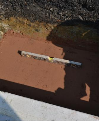
Step 2 - Use 100-150mm of either pea gravel (self-compacting) or Type 1 MOT and compact to provide a level base for precast block.
