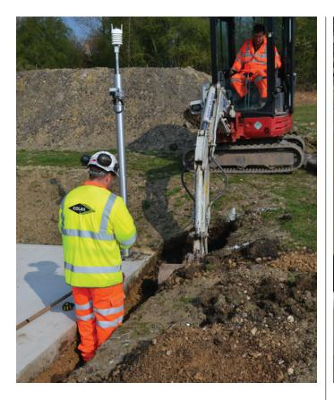
Step 1 - Excavate required foundation size for application being used, allowing 150mm (estimate) working space all the way around the block.
