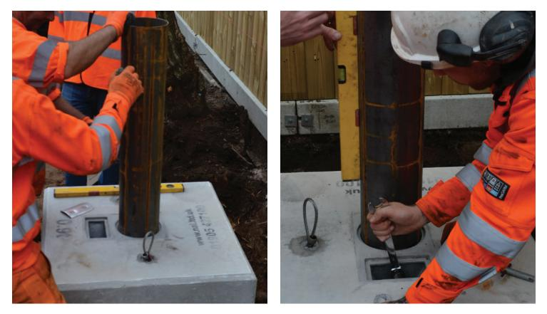
**Step 4** - Install levelling pole into the Retention Socket and tighten the locking bolts located in the side chamber of the socket to ensure levelling pole is secure. Place spirit level on levelling pole to check vertical alignment of the Precast Foundation.
