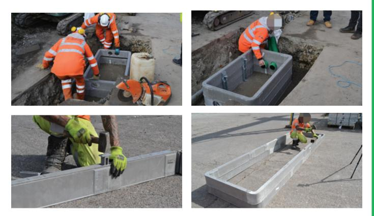
Applications: Motorway Comms, Traffic Signals, Street Lighting, Telecoms, Power, Gas, Water
