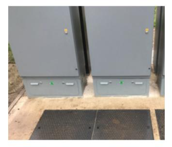
The Combined Cabinet Base is a patented system designed to simplify the installation, cabling, and maintenance of all ICEE Combined Communication Cabinets. A single ICEE Combined Cabinet provides the equivalent equipment space to three 600 type and one 609 type cabinets. This offers a large reduction in the required cabinet footprint making it ideal for sites with verge restrictions. The system is available for single or multiple cabinet sites.
